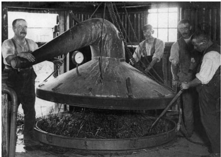
Preparing the retort for distilling mint at Miller's works, Hackbridge
