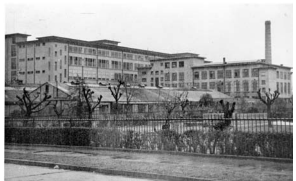
The Mullards Factory, Hackbridge
